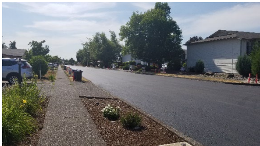
Wyatt Avenue Mill and Overlay Project 2023
