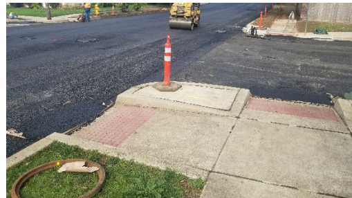
Douglas Street ADA Sidewalk Ramp 2023
